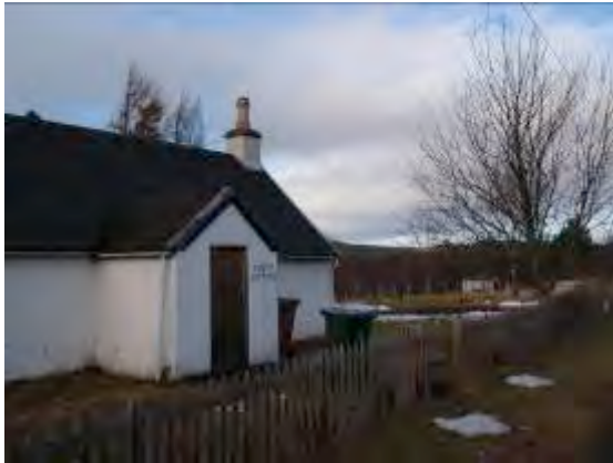
Fig. 2 Cottage from road (South)
